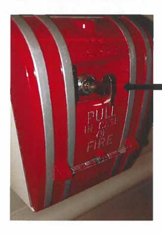
Insert key here and turn key to the right until horizontal to activate STAGE TWO ALARM
